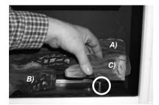
The Front Right Log front edges should be placed parallel against the front edge of the burner.
